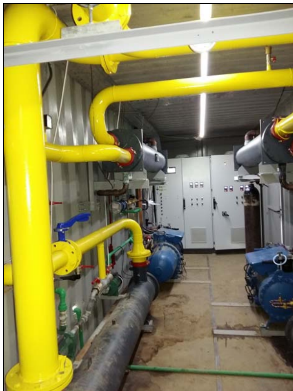
Figure 7: Two stage 1.1 MW open loop heat pump installations in a 9ha asparagus plantation in the area of Chrysoupolis (Kavala, Northern Greece).
